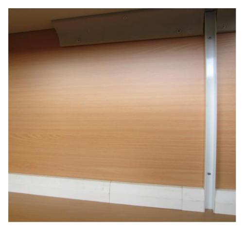
Now that the u Channel is fixed the hard bit is done. You are ready to fit the side panel. Simply slide the side panel in and fix it with screws on the inside of the U channel.
