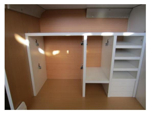
Now you are ready for the framework. Fix the return jamb in by sliding it inside the front of the side panel. You can fix it with washers and rod screws or alternatively just liquid nails. Also for additional strength you can fix the side panel to the floor with an L bracket like in the pic below.
