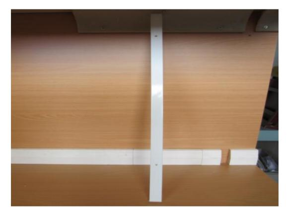
Fix the U channel to the back wall with rod screws or gyprock screws. It is a good idea to apply liquid nails at the back of the U channel for extra strength.
