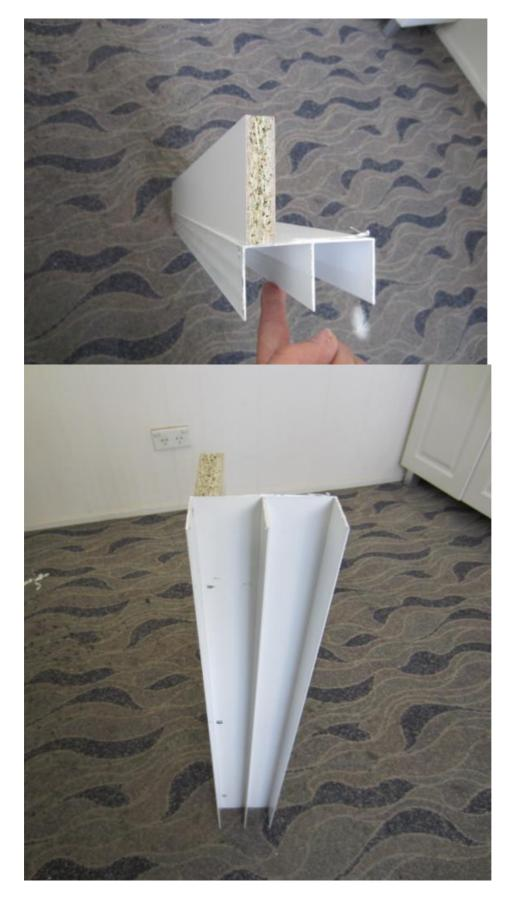
Slide the top track and bulkhead between the jambs and into the cornice slot. You may need someone to hold one side.
