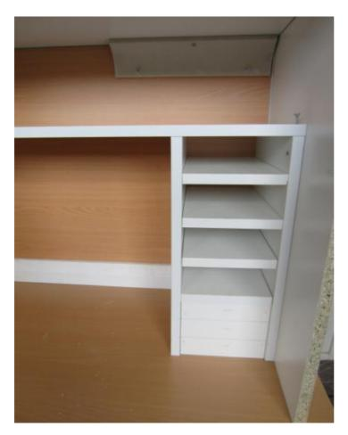
Fix the middle upright to the top shelf. Position the L brackets for the shoe shelf. Fix these using rod screws. Usually 2 screws for every bracket. Typically 300mm from the bottom of the floor.
