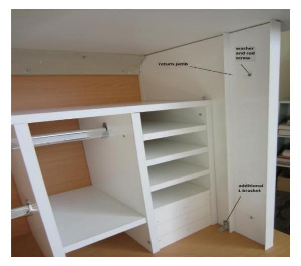
Cut an 18mm slot in the cornice 600mm from the back wall to allow the bulkhead to slide into the top. This is if the bulkhead is required.
