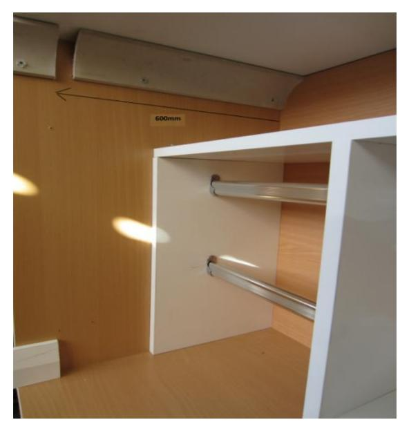
Fix the wall jamb inot the wall linig it up with the outside of the slot. Also the wall jamb needs to be leveled and sitting on the floor. Fix using rod screws, washers and liquid nails if desired.
