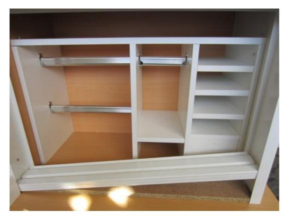
You are almost done! Place the door inside the tracks. First slide them into the top track and then drop them down onto the v groove in the bottom track. Place the first door into the back groove first. Also you can replace the missing skirting between the upright and the wall jamb on the bottom.
