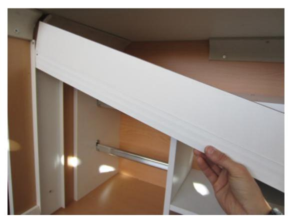
Rivet the top track into the jambs by drilling with 3 or 3.5mm drill bit. Measure and cut the floor batten and sot it into place between the jambs.
