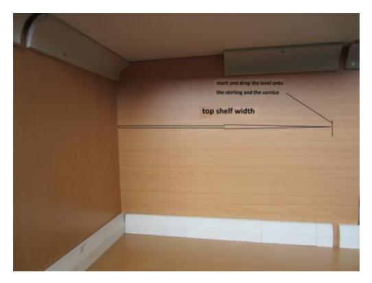
Cut The skirting out 600 mm from the back wall so that it can accommodate the side upright. Note: If there are existing skirting boards all the uprights need to be cut out on the bottom to sit past the skirting boards.
