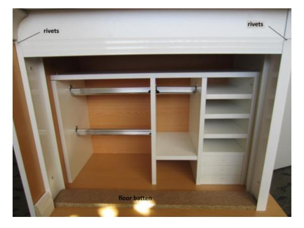
Put the bottom track in. Rivet the bottom track same as the top to the jambs. Please note usually it is not neccesarry to fix the bottom track to the floor as the rivets and the weight of the droos hold it down.
