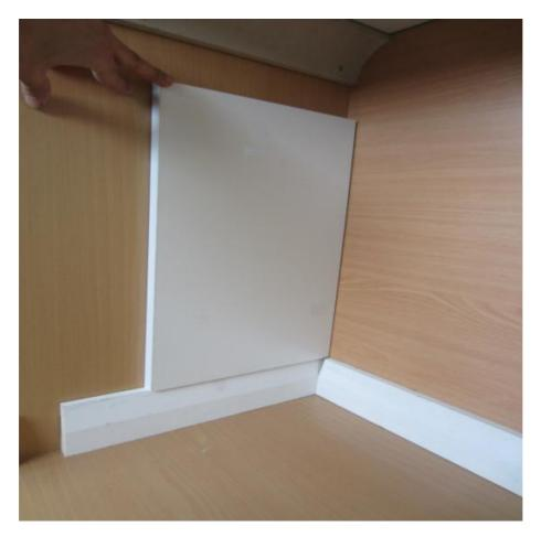
Drill The U channel on the back and on the side with a 2 or 3mm drill bit. 3-or 4 holes.
