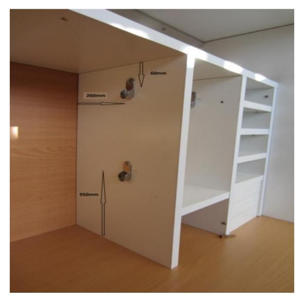
Now with all the rod supports in place you are ready for rods. Just cut measure between the rod supports and cut them to the size. Place them inside the rod supports.
